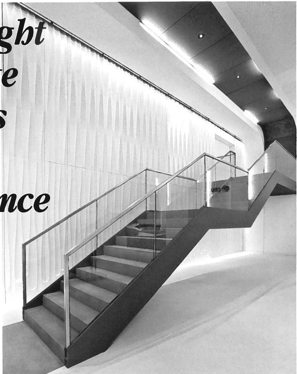
A 156m 2 massive curtain of lightweight concrete with optic, acoustic and biological effects.
